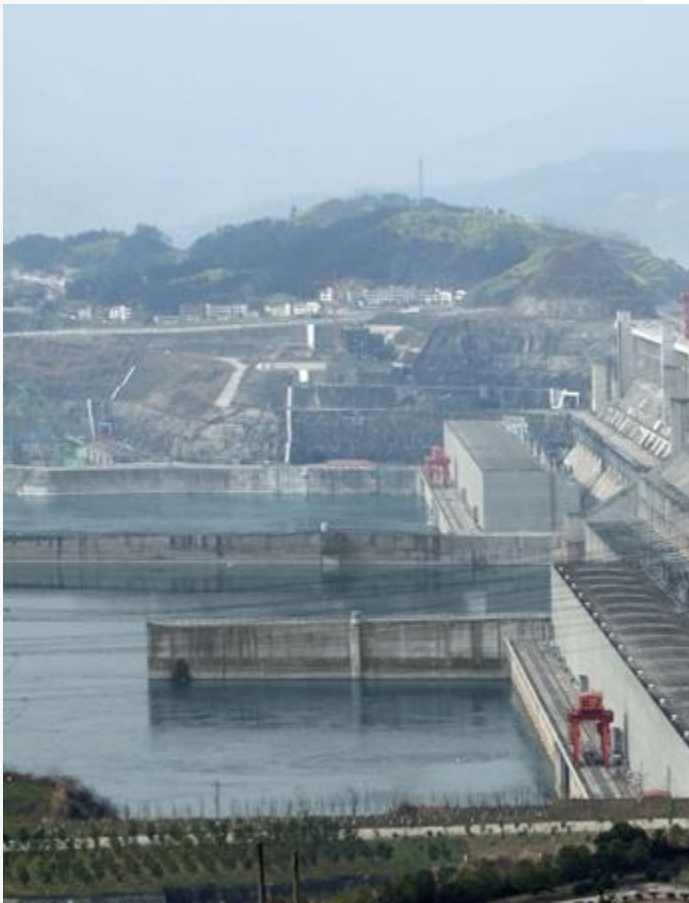
Image of the Three Gorges Dam: The world's largest hydroelectric power station
